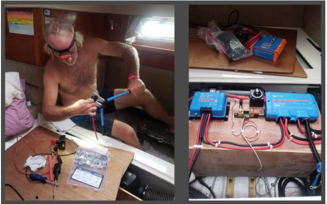
Hot work in Panama prepping for the new batteries
